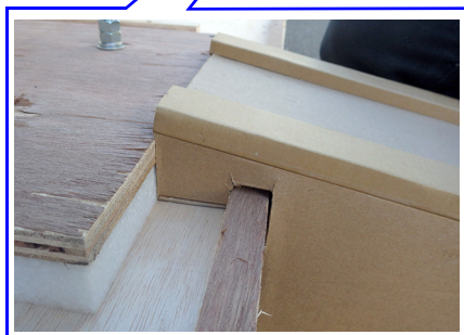
Figure 1-40. Setting the ramps
